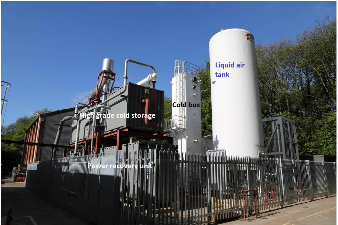
292 Figure 7. 350kW/2.5MWh Liquid air energy storage pilot plant at the University of Birmingham, UK.
